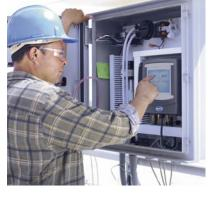
A large color touchscreen lets operators observe system status quickly. Parameters can be adjusted easily when processes change.
