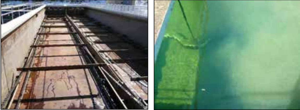
Figure 26: Rectangular clarifier sludge removal system Left, basin with flight and chain sludge removal system. Horizontal scrapers move settled sludge to a collection trough. Right, as water passes through a clarifier, settling progresses, one sees the floc cloud ending before the water reaches the end of the clarifier. Photos by author.
