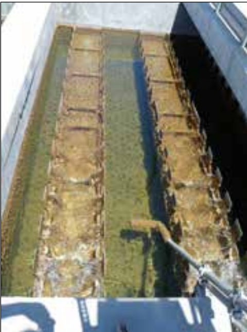
Figure 32: Tube Settlers enhance settling
