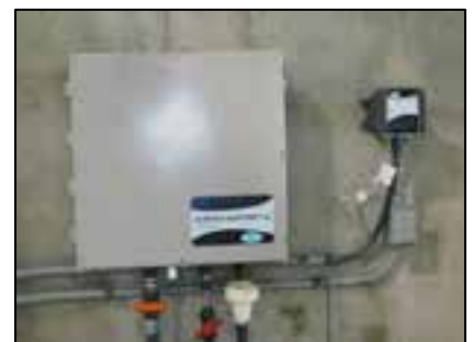
Figure 42: Turbidity and suspended solids monitoring for clarifier effluent
