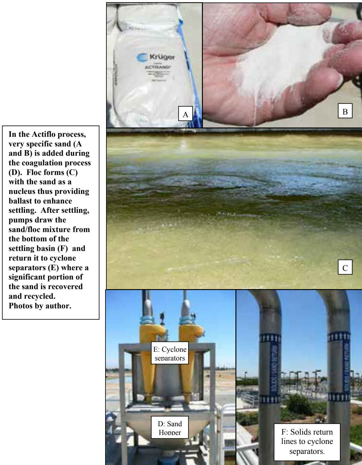
Figure 16: Actiflo process for ballasted flocculation
